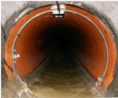
Figure 2. Flow measurement using the velocity-area method
