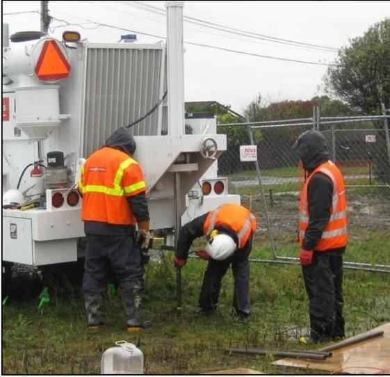
(a) Installing 2D velocity transducers (geophones) and pore pressure transducers (PPTs) with the hydraulic ram on the back of T-Rex.
