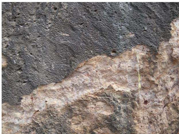
Fig. 4. Surface crust with Ca-oxalate in volcanic stone of ashlar from the abside of St. Antioco di Bisarcio
