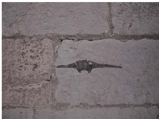
Fig. 3. Wall facing of the transept S of the Santa Maria Assunta Cathedral at Pisa, showing the presence of SVL limestones with a typical black flint.
