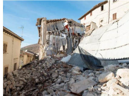
Fig. 3. The collapsed church in October 2016.
