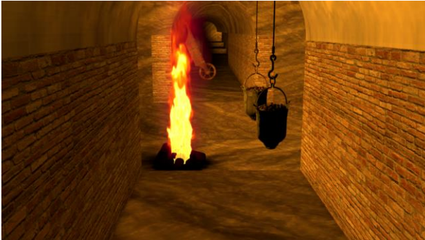
Fig. 4. Virtual reconstruction of the Roman emissary under construction. The buckets are a reproduction of the ones found during Torlonia's excavations. The bucket is now part of the Torlonia Collection of Antiquities of the Fucino area, hosted in Celano, Museo d'Arte Sacra della Marsica e della Collezione Torlonia di Antichità del Fucino, Italy. The wheelbarrows are inspired by De Re Metallica.
