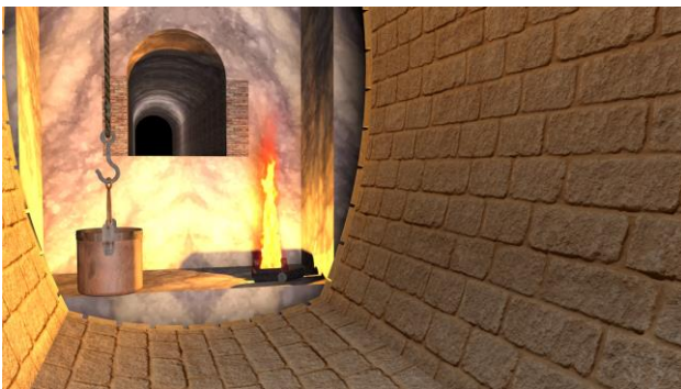
Fig. 8. This picture confronts the Torlonia emissary with the Roman tunnel, represented near one of the roman well. It can be seen the difference in heights between the two tunnels and the width of the respective sections.
