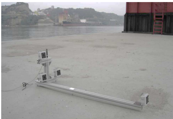
Fig. 2. Active targets on the south tower foundation
