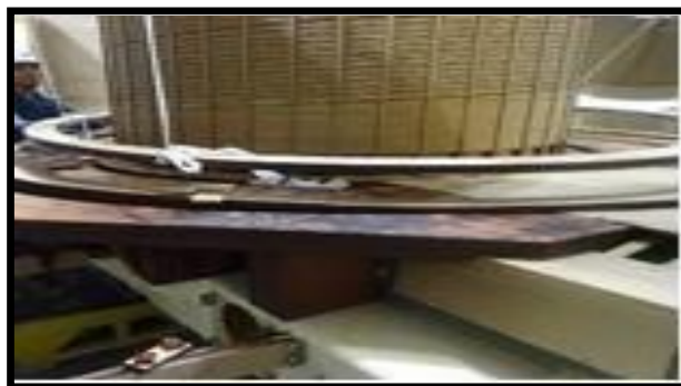
Fig-7: Series + Common winding during dismantling.
